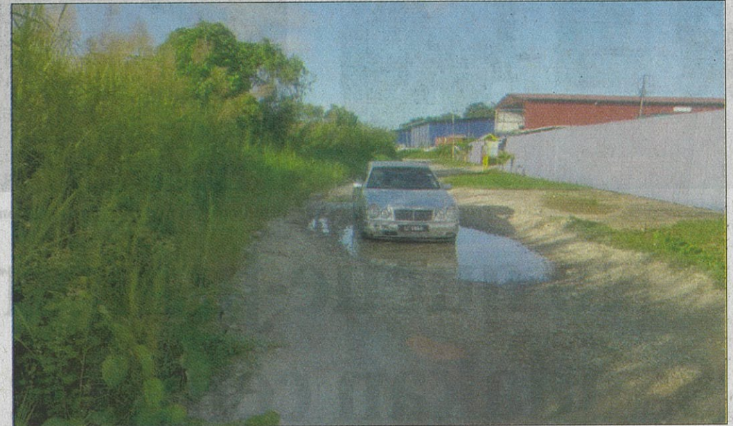
The sorry state of the road to the crematorium.
